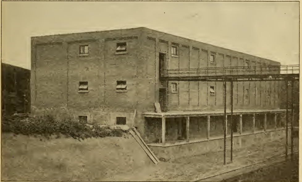
The A. I. Root Company's Fireproof Warehouse, 148 x 48, three stories, with loading-platform and steel bridge connecting old Warehouse on the south.
